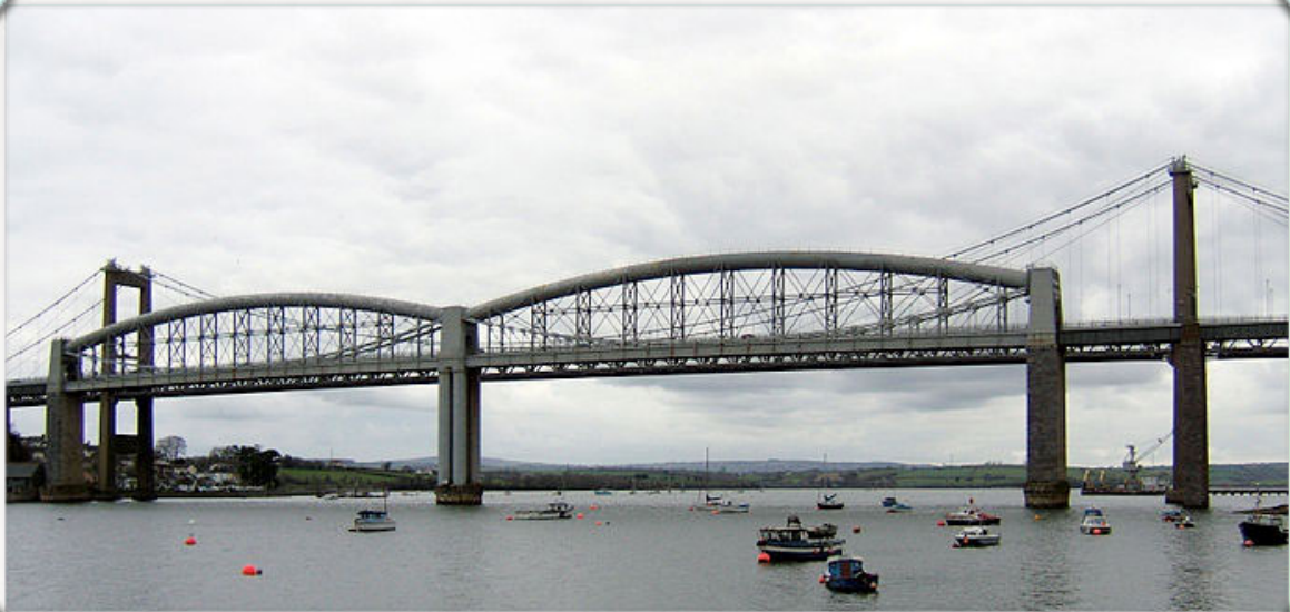
The Royal Albert Bridge
