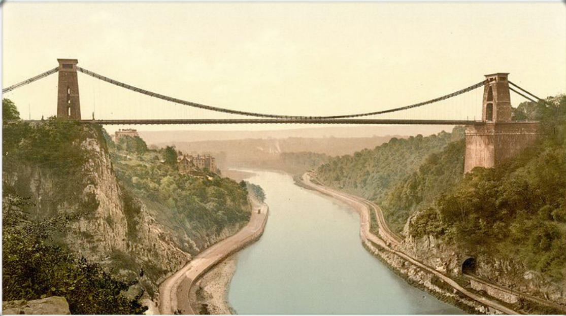
Clifton Suspension Bridge
